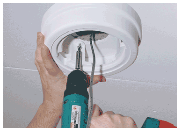
Step 1: Secure Housing to Mounting Surface
