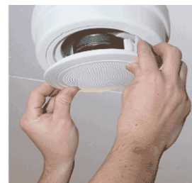
Step 3: Fit Speaker to Housing
