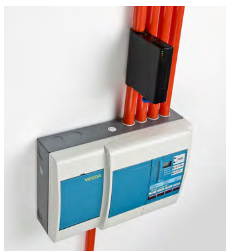
VESDA ECO installed on sampling pipe
