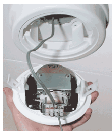
Step 2: Terminate Cable
