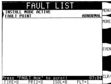
Figure 8-3. Fault List Now With Only a Single Install Mode Fault
