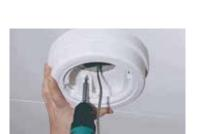
Step 1: Secure Housing to Mounting Surface
