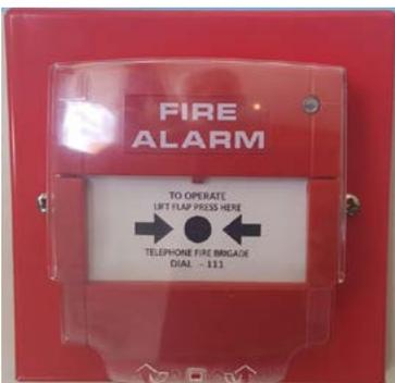
The kit makes use of the existing 1841 surface-mount back box or flush-mounting box so that the new MCP can be fitted without disturbing the existing cabling, fixtures, and paintwork. The colour and outside dimensions of the adaptor plate match the 1841 MCP.
