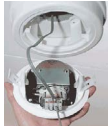
Step 2: Terminate Cable
