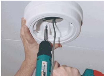
Step 1: Secure Housing to Mounting Surface
