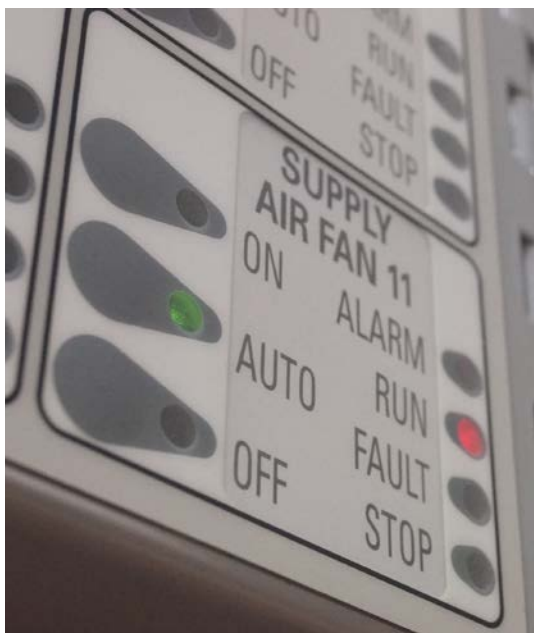
FIG 2. Each control includes labelling space for the control, push buttons, and the 4 LEDs. Up to 5 Fan Control Doors can be fitted to the FP1084 15U Cabinet. The standard 15U MX1 can accommodate up to 3 FP1056 Fan Control Doors.
