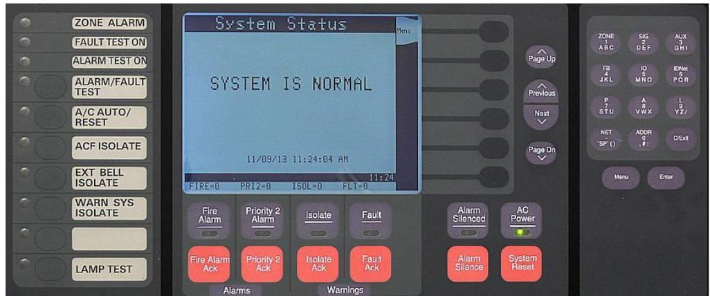
**Figure 2-3. InfoAlarm Operator Interface**
