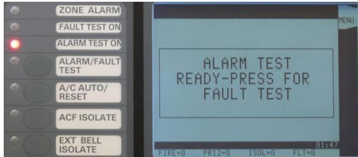
Figure 5-1. Ready for Zone Alarm Test
