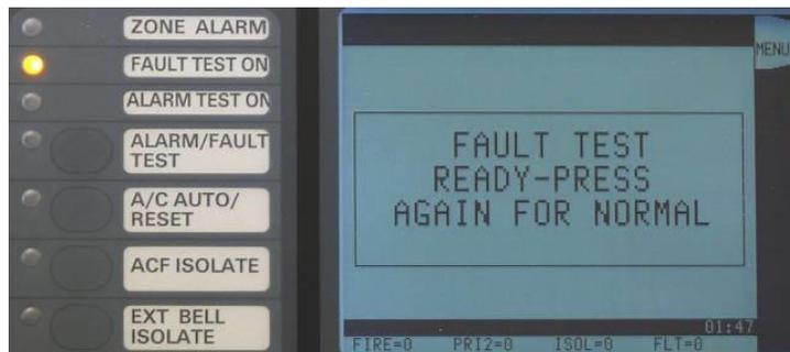
Figure 5-2. Ready for Zone Fault Test
