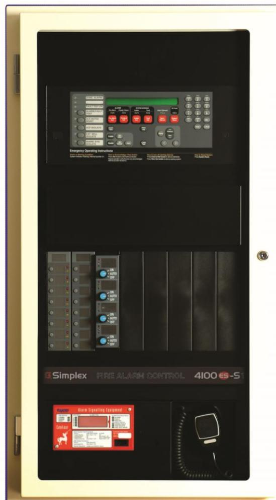
The 4100ES-S1 comes in a 21U cabinet with external dimensions 1050 x 575 x 280mm (H x W x D), with a cream wrinkle finish.
