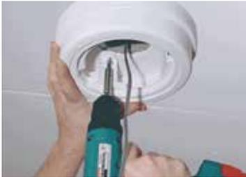
Step 1: Secure Housing to Mounting Surface
