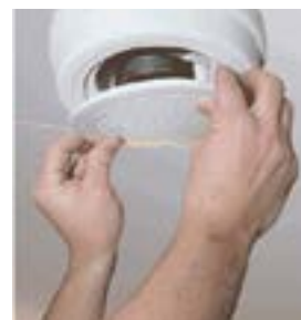
Step 3: Fit Speaker to Housing
