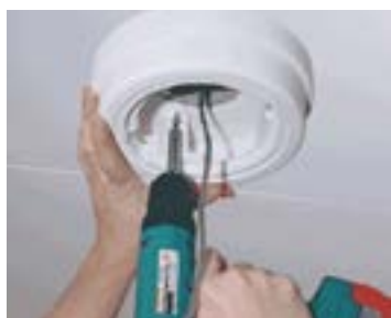
Step 1: Secure Housing to Mounting Surface
