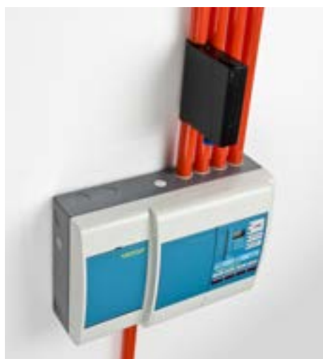
VESDA ECO installed on sampling pipe
