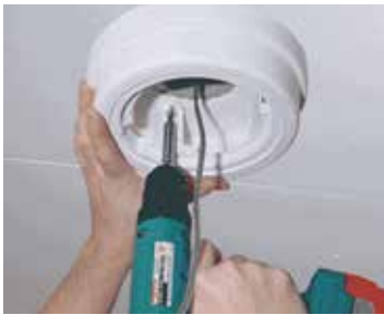
Step 1: Secure Housing to Mounting Surface
