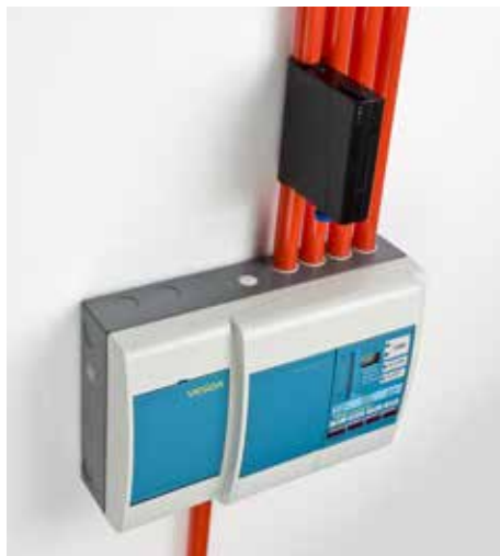
VESDA ECO installed on sampling pipe
