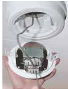
Step 2: Terminate Cable
