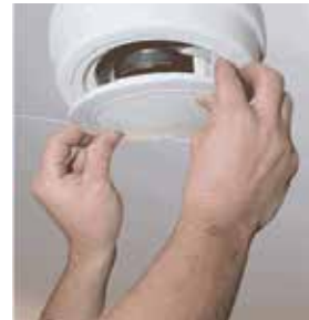
Step 3: Fit Speaker to Housing
